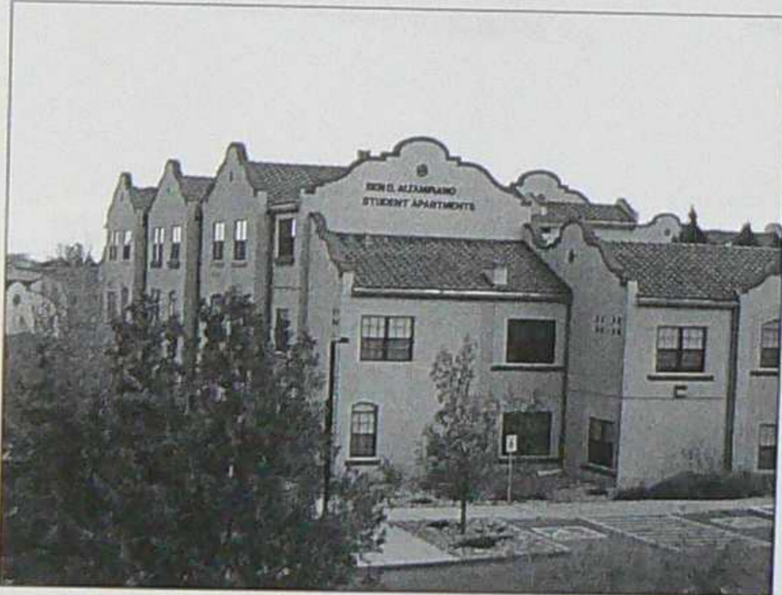
Ben D. Altimirano Student Apartments Completed 2000
