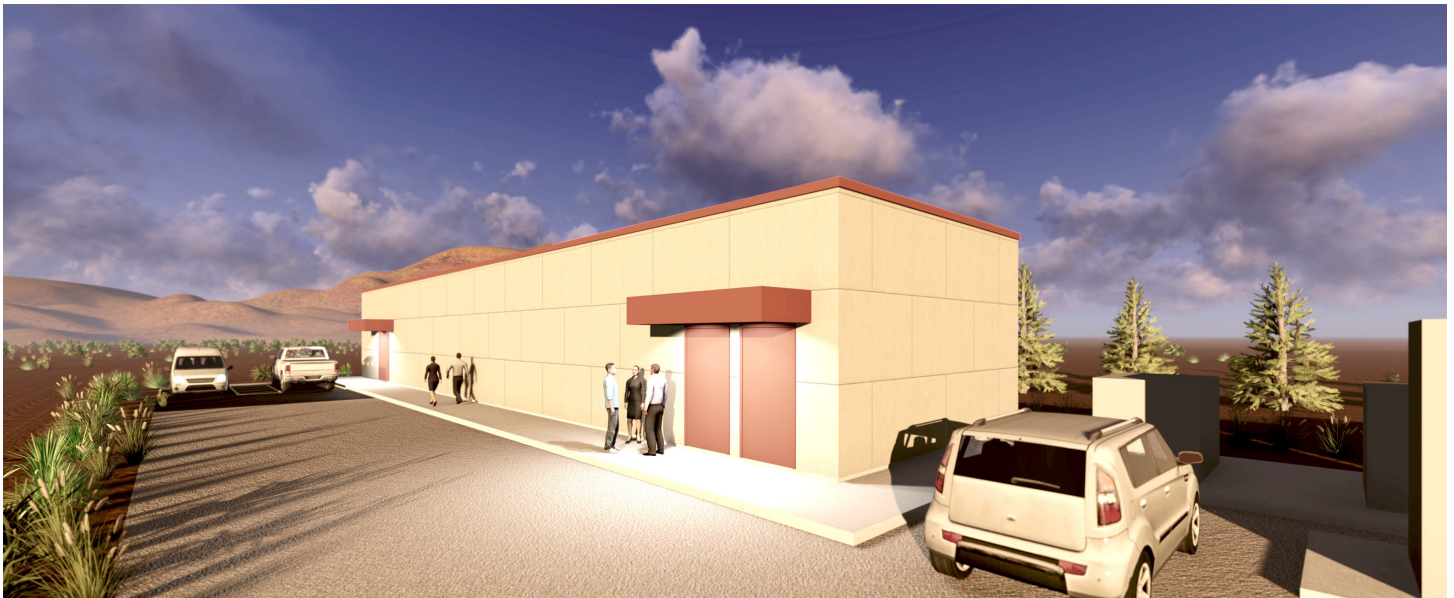
Data Center, to be completed in early 2018
